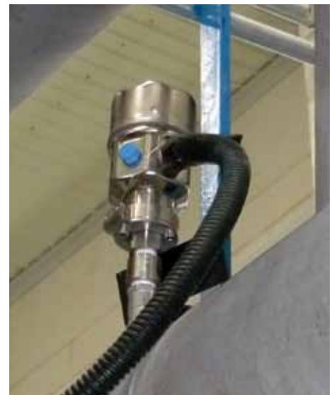
Accurate pressure measurement in a membrane system
