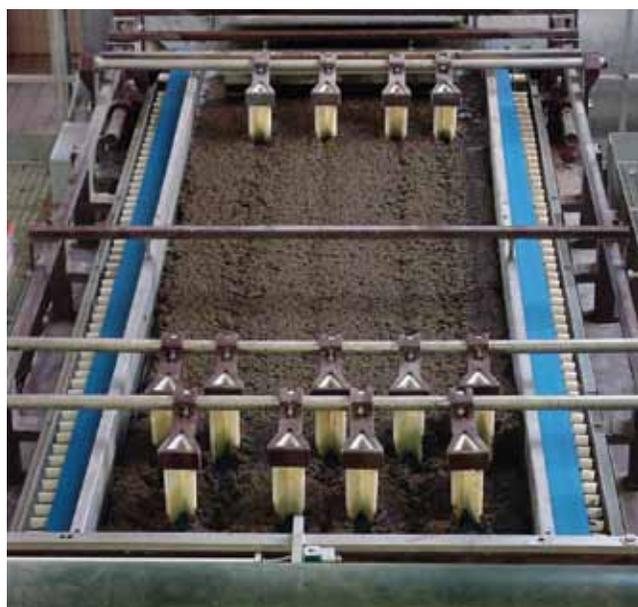
Belt filter in a sewage facility for sludge dewatering
