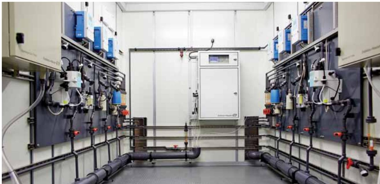
Container solution of Endress+Hauser for efficient water management in production and auxiliary circuits
