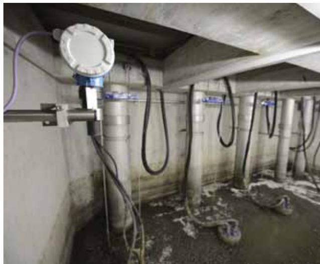
Dependable level measurement in the extensive sewerage system
