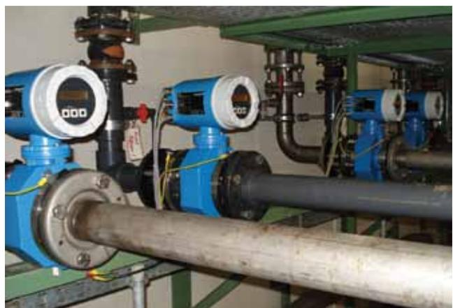
Reliable monitoring of flow rates with Promag electromagnetic flowmeter
